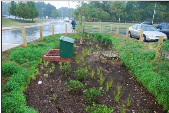
Construction at ACC was conducted over the summer months of 2011. Construction was complete on September 9, 2011. This project consisted of two innovative bioretention areas in the school's parking lot and a 4,900-gallon water storage cistern.
